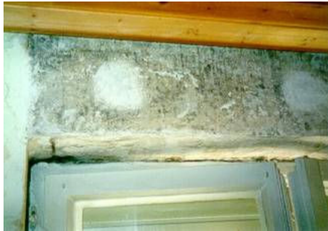
Figure 4: Mould found at the dewpoint after removal of drylining Image courtesy of the Fraunhofer Institute, IBP Holzkirchen
